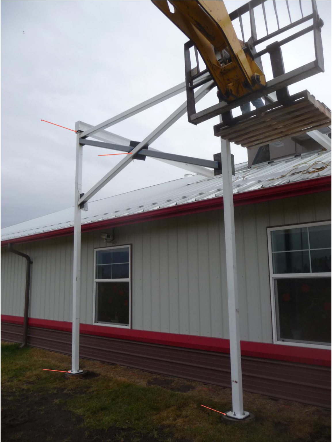
KELLETT Vibration Isolation Pads installed at multiple locations in Rack.
